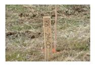
Reestablish the catch point if the slope stake is accidentally destroyed or moved during construction. If a guinea is missing and the slope stake remains, the contractor and the engineering personnel will know it is not a catch point.
